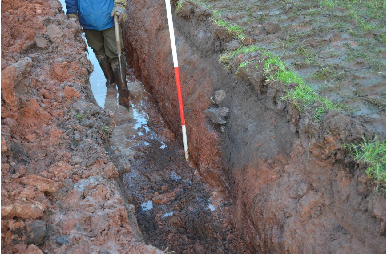
11. Ditch and field drain at NY 56873 37195, east section (the ranging pole is in the same location as in photo 14).
